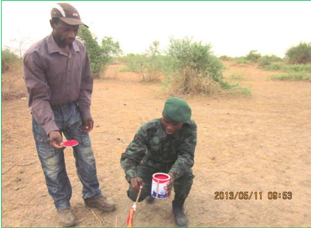
The work of clearing and staking site
